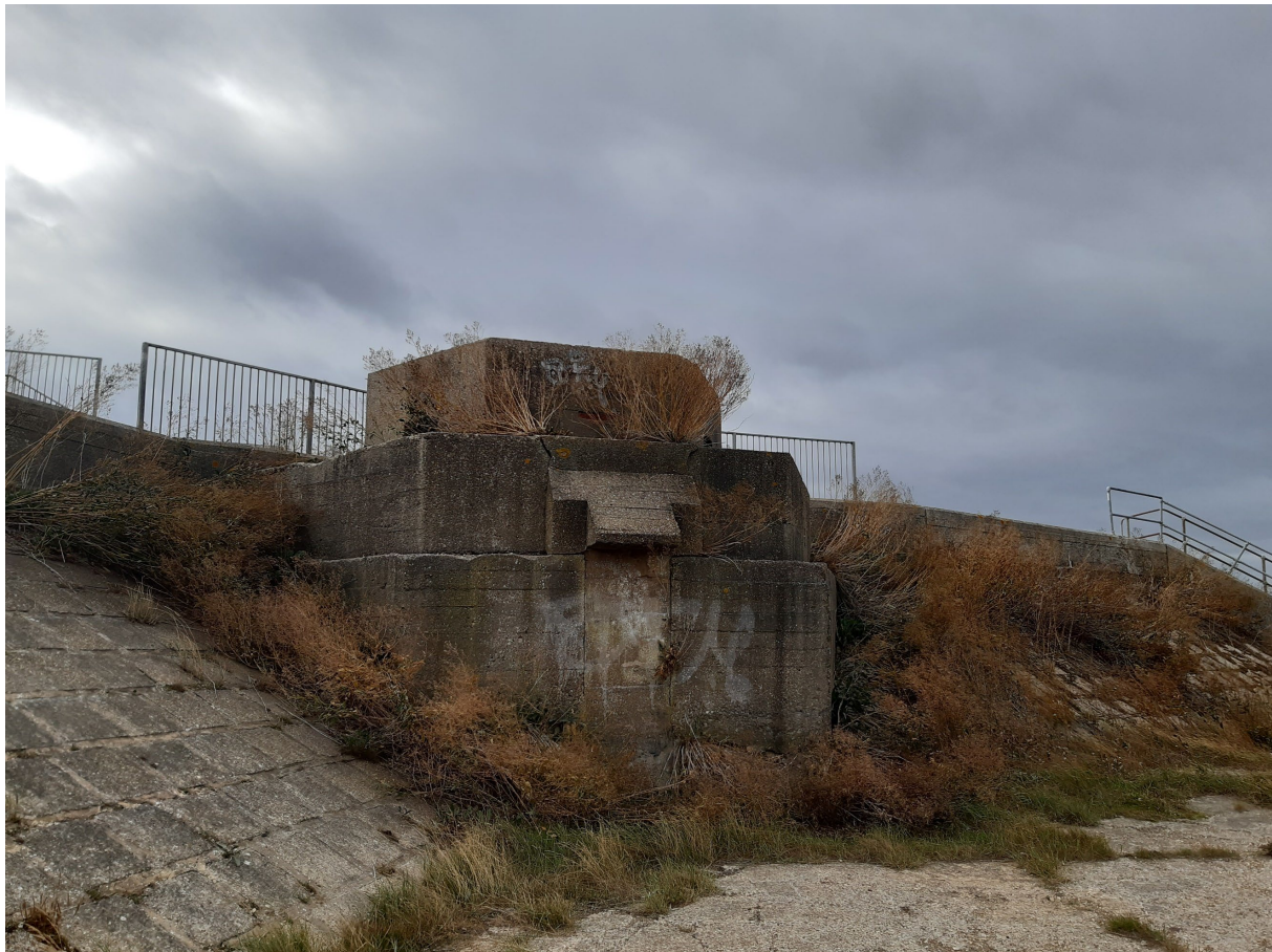
Plate 2 View of Pillbox at Sandy Point from the north-east
