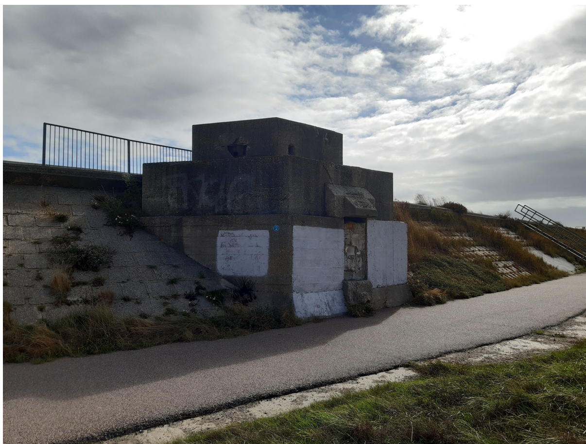
Plate 3 View of Pillbox east of Chevaux de Frise Point, looking south
