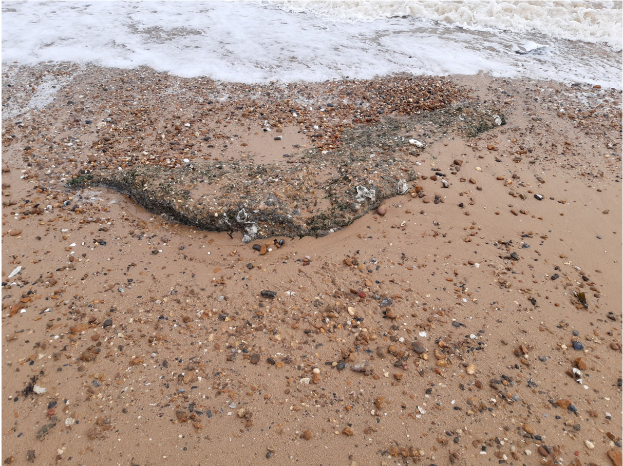
Plate 6 Remains of Pillbox on the beach, looking south south-west
