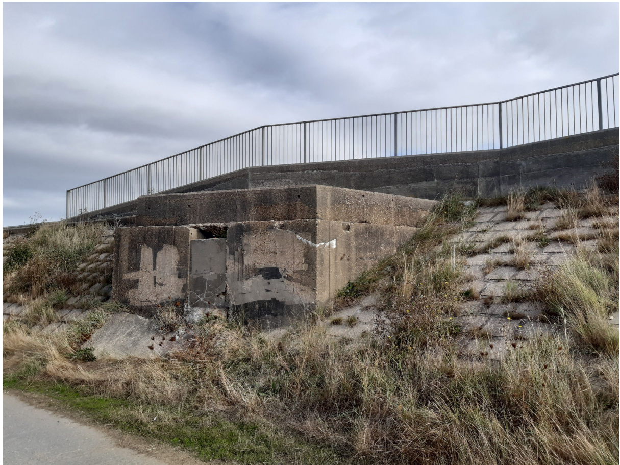
Plate 4 View of Pillbox at Chevaux de Frise Point, looking east
